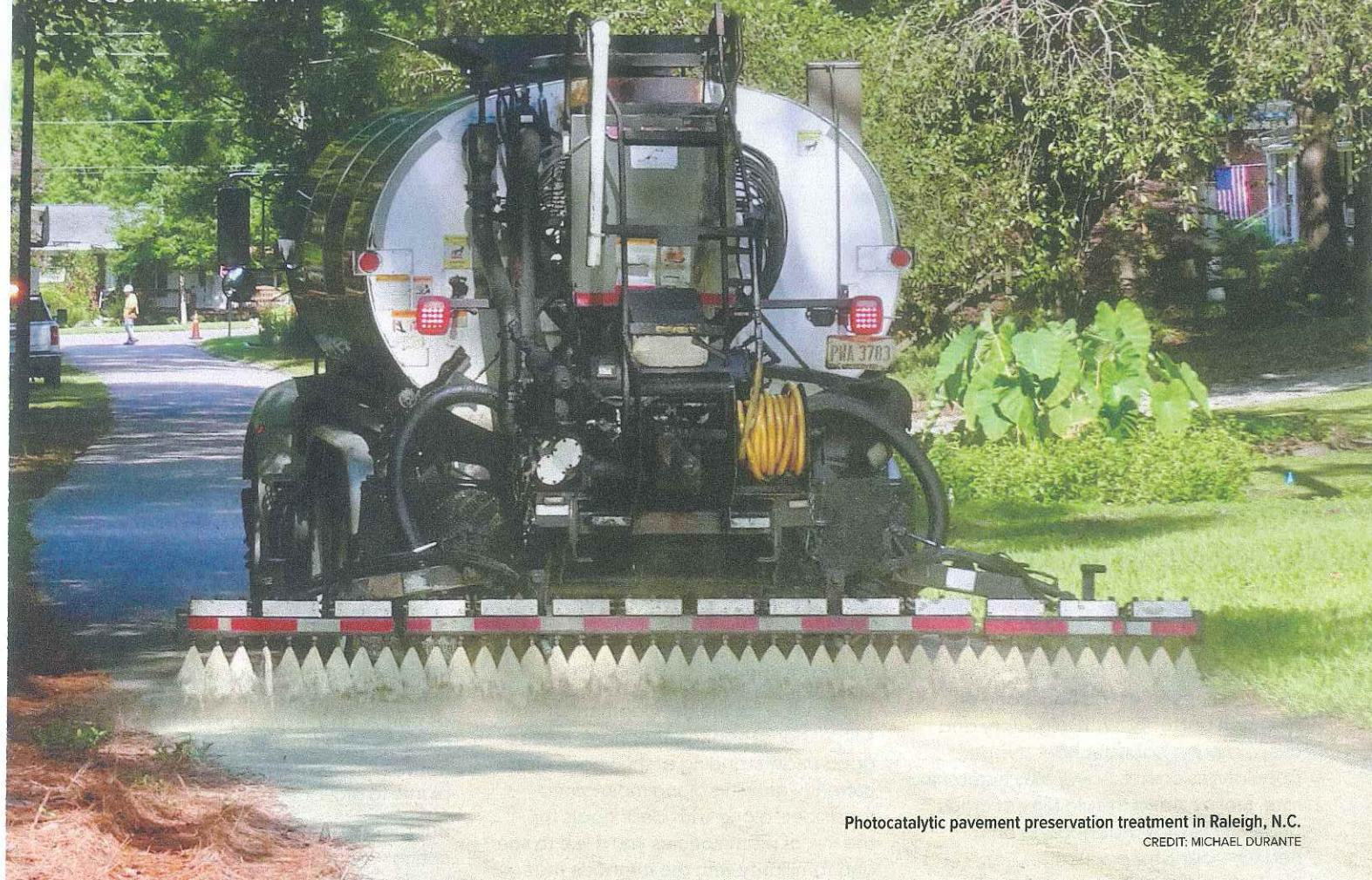
Photocatalytic pavement preservation treatment in Raleigh, N.C.
